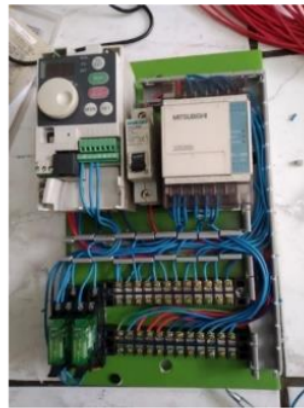
Figure 2 The process of installing power and power cables
