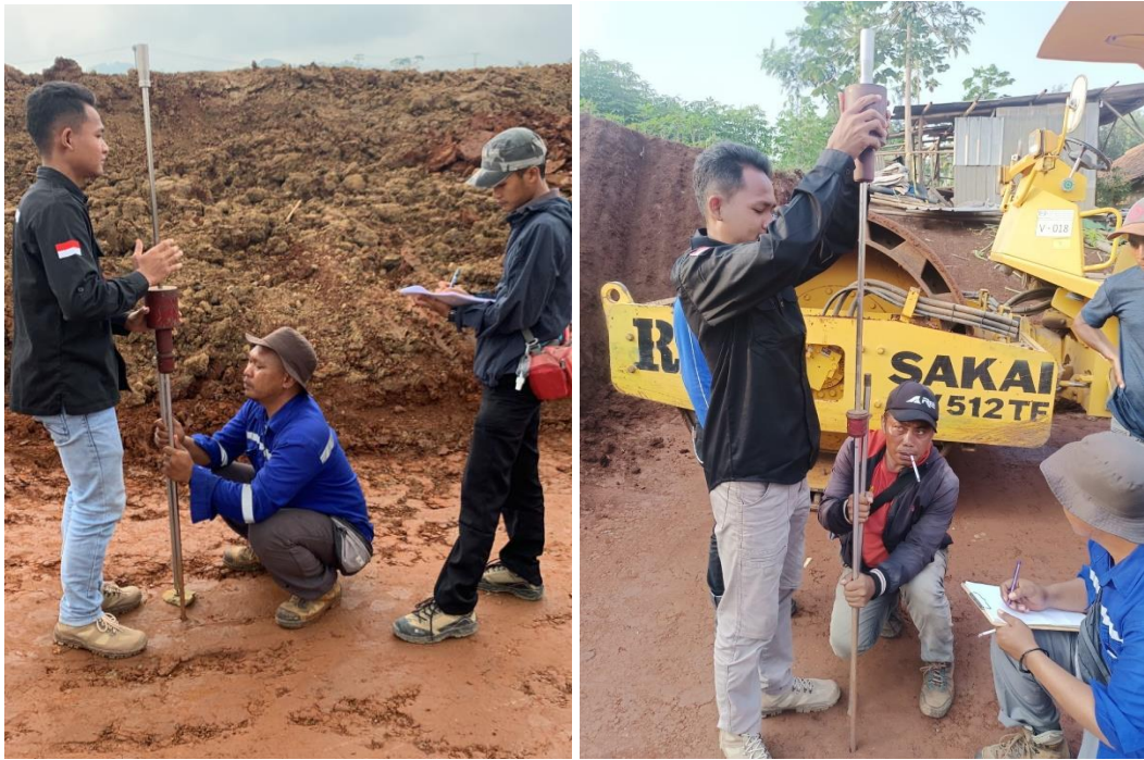
Gambar 1 Proses Uji Dynamic Cone Penetrometer (DCP)
